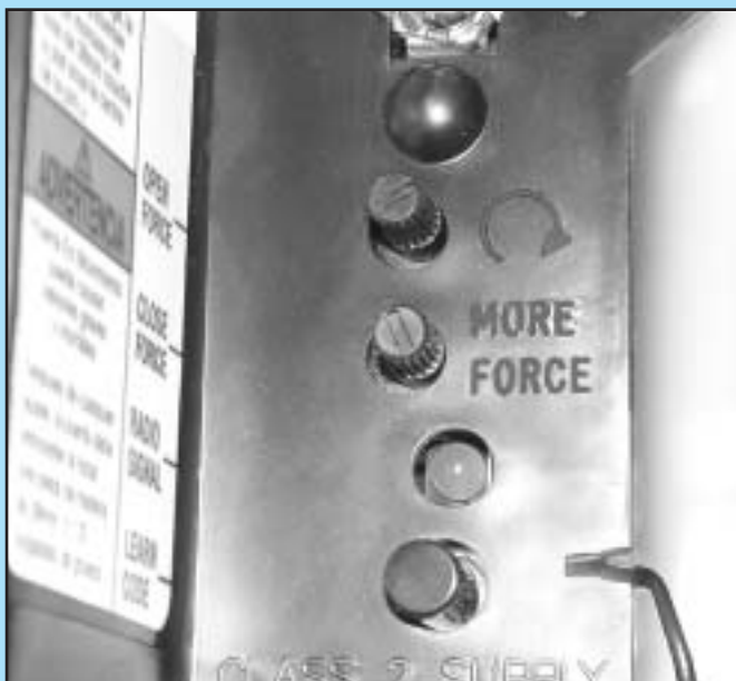
FIG. 7-1 Force adjustment screws.
