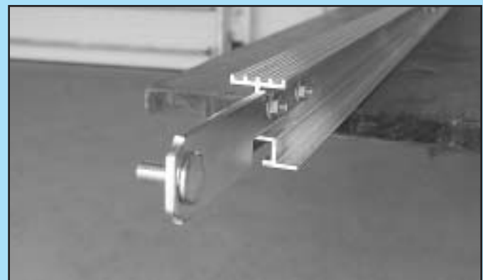
FIG. 1-4 Attach rail strap.
