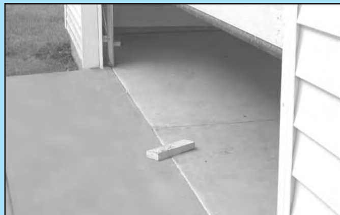
FIG. 6-5 2 x 4 under center of door opening.
